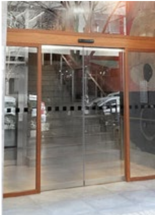
Resistance Leaf with top and bottom profile and 20 mm glass.
