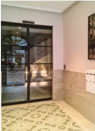
Robustness Leaf with full framed profile and 30 mm glass.
